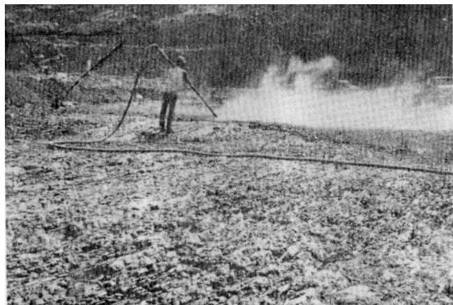
Figure 3-1. Final foundation cleaning using compressed air, DeGray Dam, Arkansas
