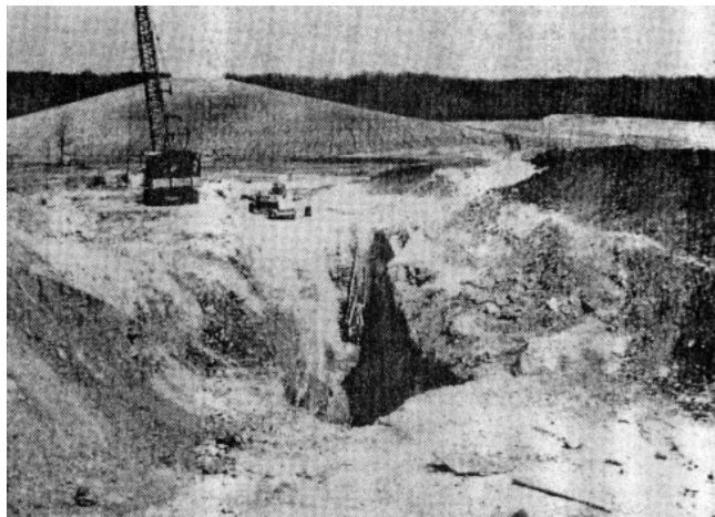
Figure 3-6. Solution channel, Mississinewa Dam, Indiana
