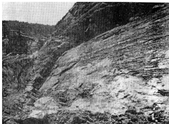
Figure 3-7. Abutment overhang, DeGray Dam, Arkansas
