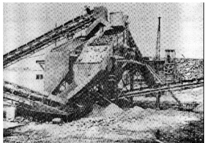
Figure 4-5. Vibrating screen separating plant
