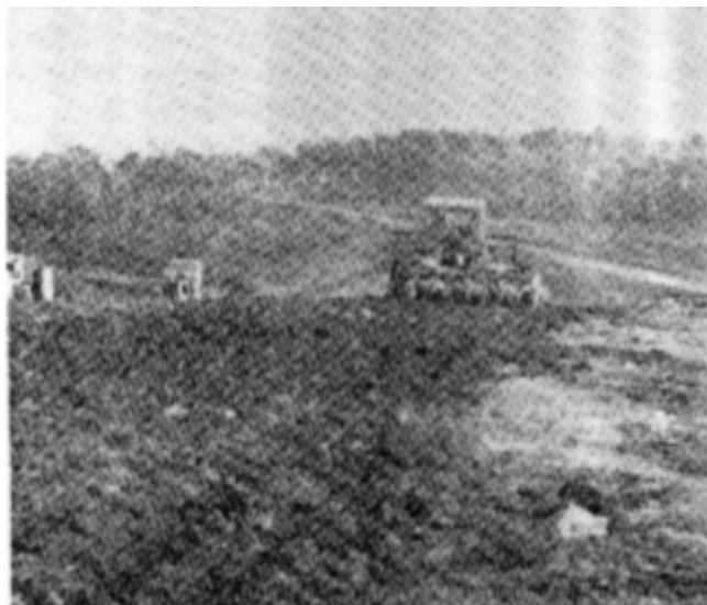
Figure 5-4. 36-in.-diam disk towed by D-8 tractor at DeGray Dam, Arkansas
