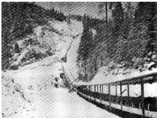
Figure 4-4. Belt conveyor system
